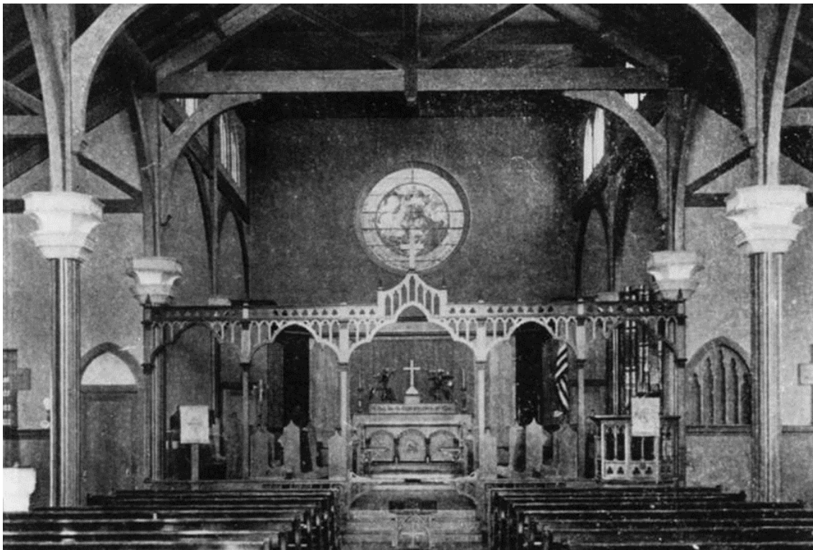
Figure 13. Sanctuary addition with exposed timber roof, circa 1915; note wooden balustrade (since removed) and modified column capitals (Security Pacific National Bank Collection/Los Angeles Public Library)
