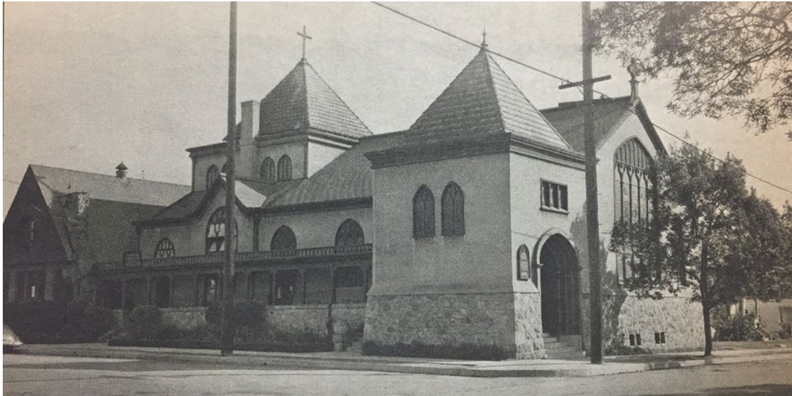
Figure 13. Sanctuary addition with exposed timber roof, circa 1915; note wooden balustrade (since removed) and modified column capitals (Security Pacific National Bank Collection/Los Angeles Public Library)
